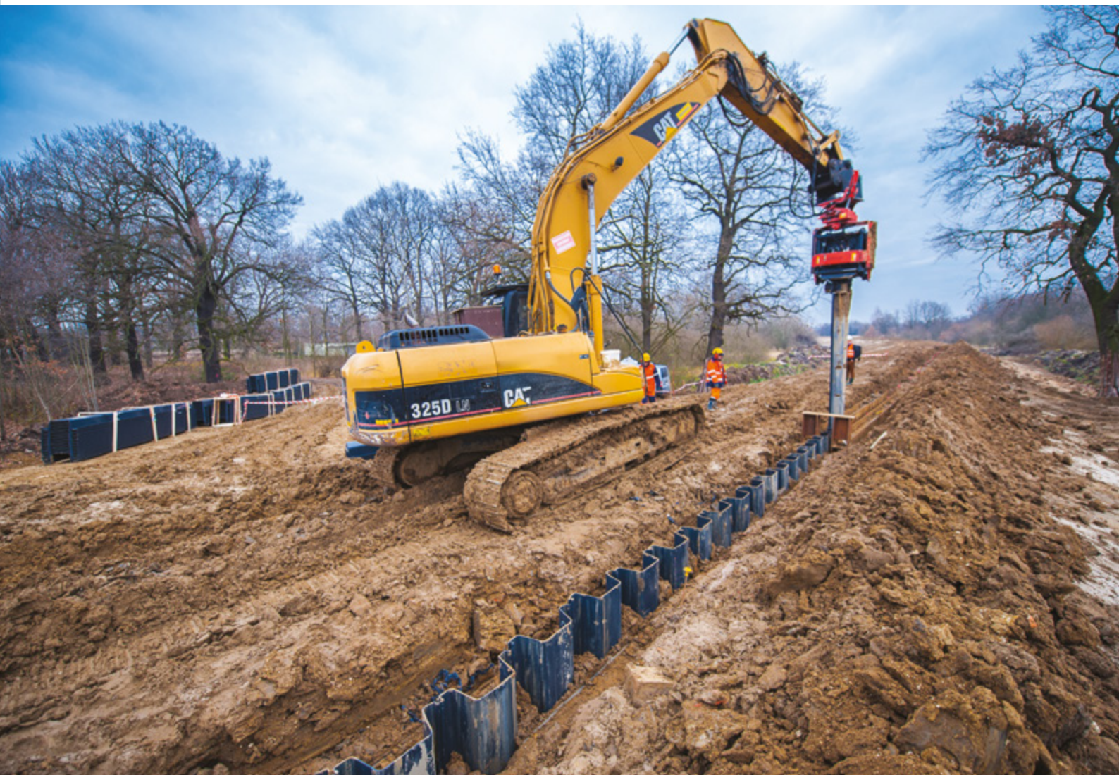
Vinyl sheet piling used to reinforce flood-walls.
